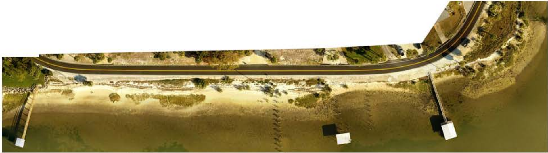
C. Airport Rd. – Present Condition
